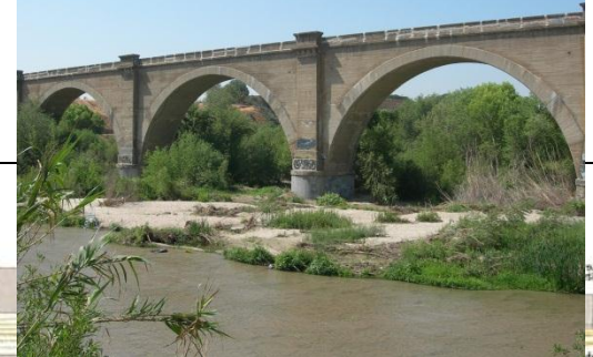
Santa Ana River Bridge
